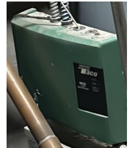
Hydronic systems External zone valve control
